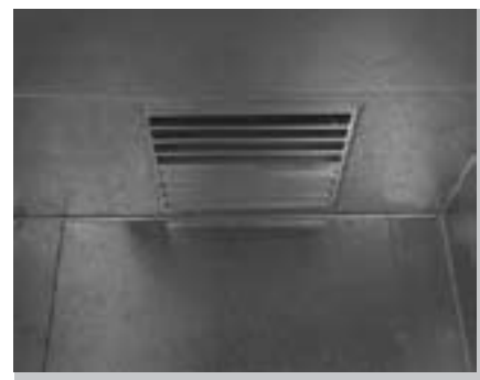
The PRO 3 evaporator grill sits flush in the ceiling of the indoor cooler or freezer
